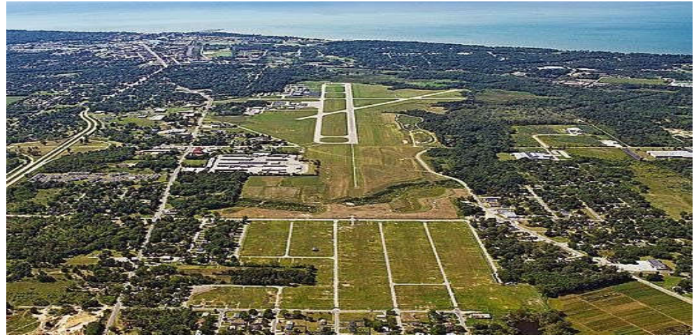
Runway 10/28: 6005 feet long by 100 feet wide
