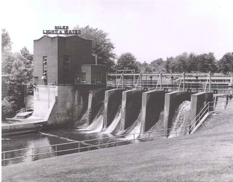
Looking west at dam and powerhouse. Date unknown (after 1928)
