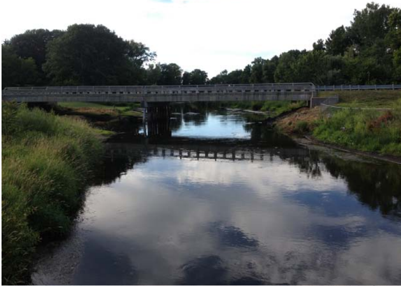
Pucker Street Bridge. Existing
