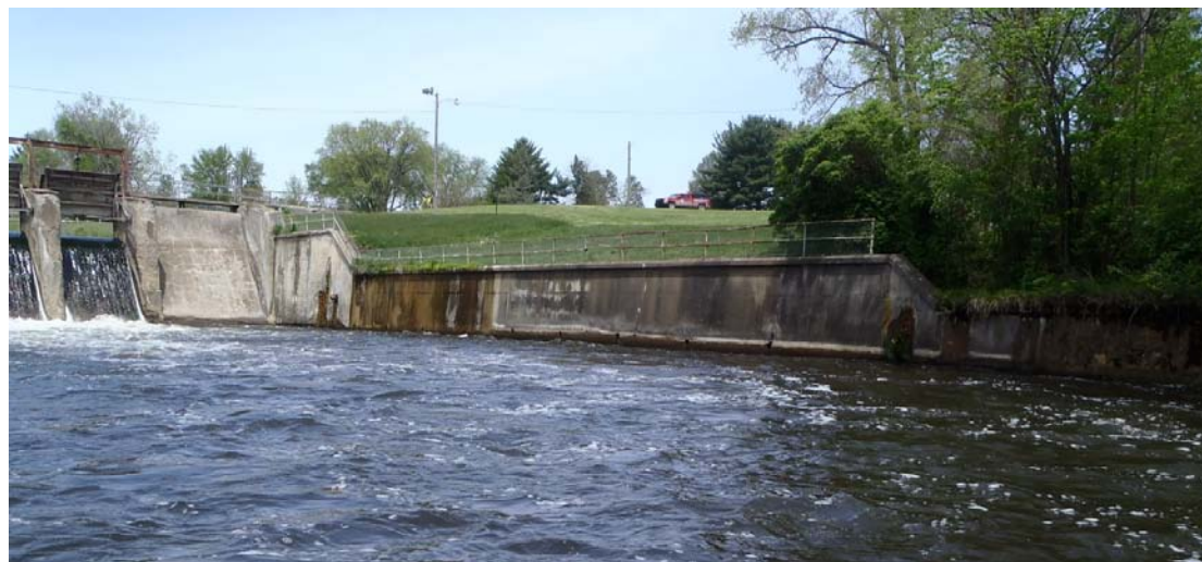
Looking upstream at east concrete wall and spillway. Existing
