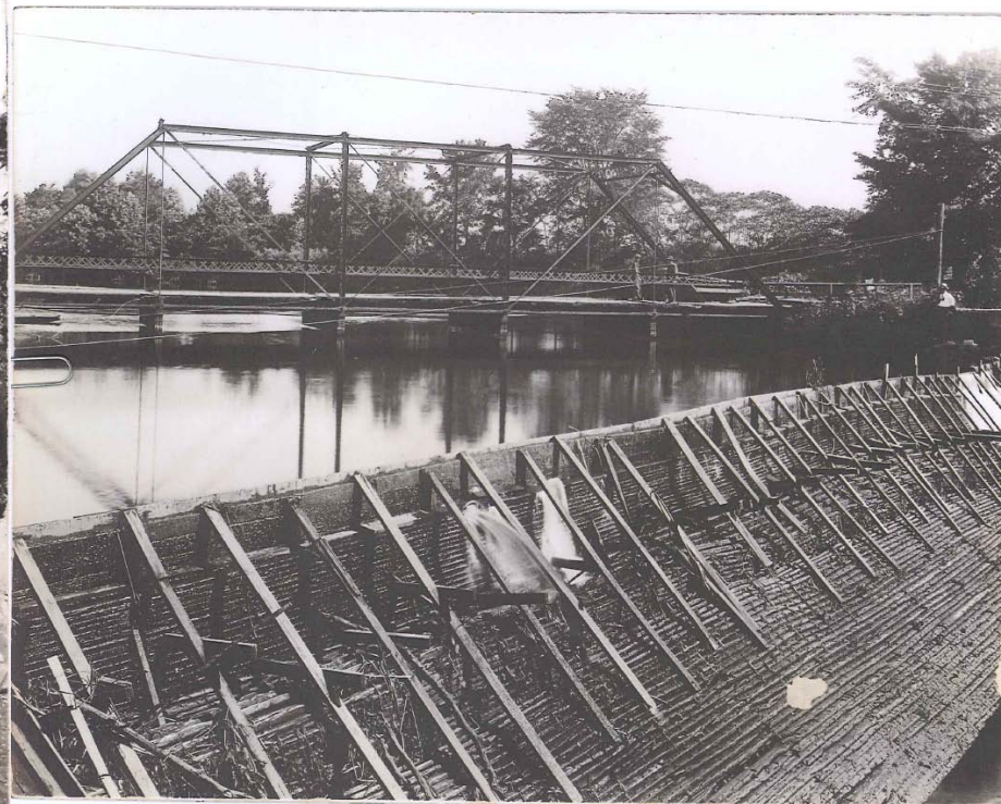
Old dam and Pucker Street Bridge. 1924
