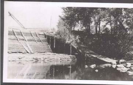
Looking east at dam, apron and fish ladder.
