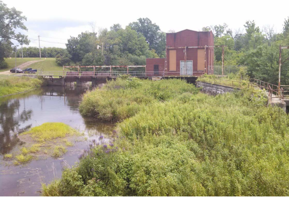
Looking downstream (south) at power house and dam. Existing
