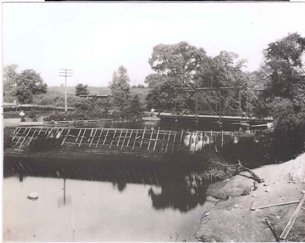
Old dam and Pucker Street Bridge. August 1928
