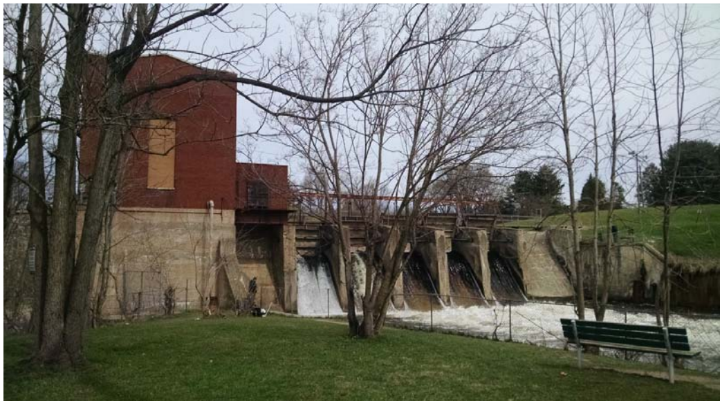
Looking upstream at dam and powerhouse. Existing
