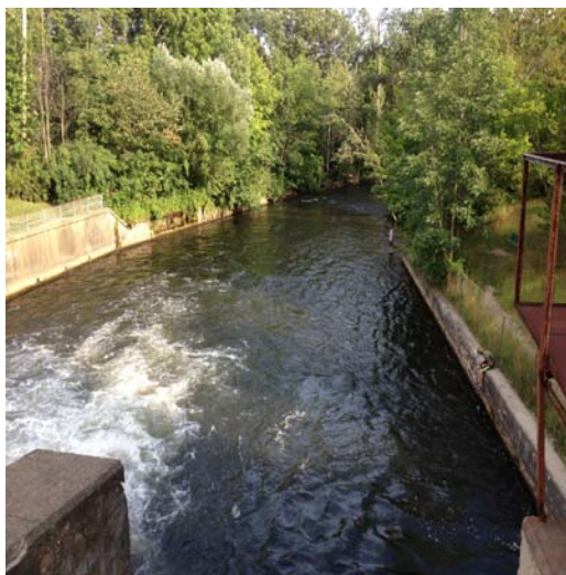
Looking downstream at east and west concrete walls. Existing
