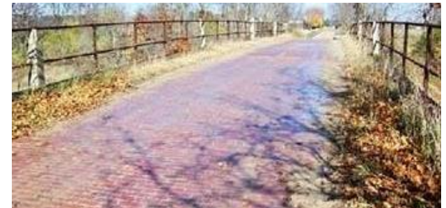
The Thomson Road Bridge, constructed in 1919, spans the now abandoned Michigan Central Railroad switchyard. This bridge is included on the National Register of Historic Places, as an early testament to T-beam construction and boasts a unique brick deck, a feature seldom found in similar structures.
