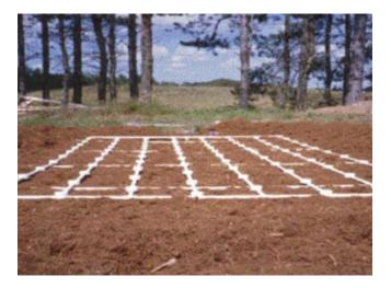
*Placement of a pipe distribution network in a peat filter* Source: University of Minnesota, NERC
