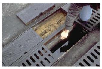
*Linear perimeter filter in trench drain* Source: Georgia Stormwater BMP Manual
