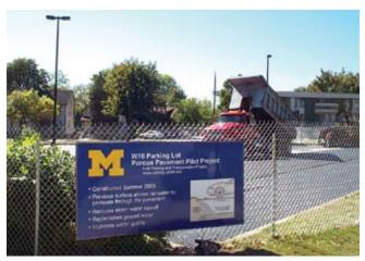
Figure 7.35 **Porous asphalt on open-graded stone subbase**
