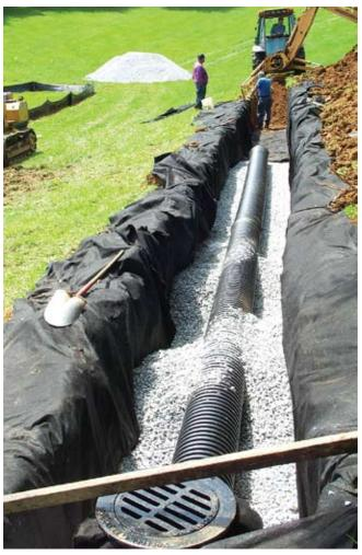
Infiltration trench with geotextile
