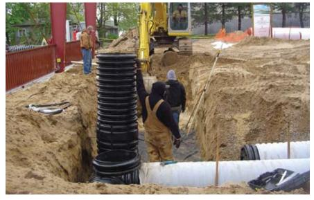
Subsurface Infiltration Source: JFNew
