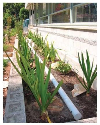
Perforated pipe used for inflow/distribution in a stormwater planter box Source: www.wsud.org
