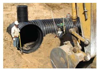
*Subsurface infiltration bed* Source: Driesenga & Associates, Inc.
