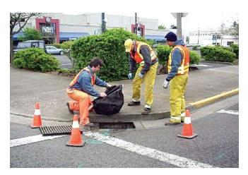
Installing a bag type catch basin insert When filled with sediment, a machine such as a bobcat or backhoe may be needed to lift the bag from the catch basin. Source: Pennsylvania Stormwater BMP Manual, 2004
