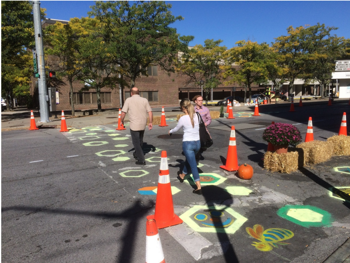
Figure 7 Temporary Pedestrian Crossing - Poughkeepsie, NY
