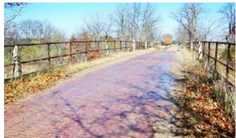
(D) The Thomson Road Bridge, rated a 4, was built in 1919 over the now abandoned Michigan Central Railroad switchyard. It's historically noteworthy as a very early example of T-beam construction and it has a brick deck—which is rare. It's listed on the National Register of Historic Places.
