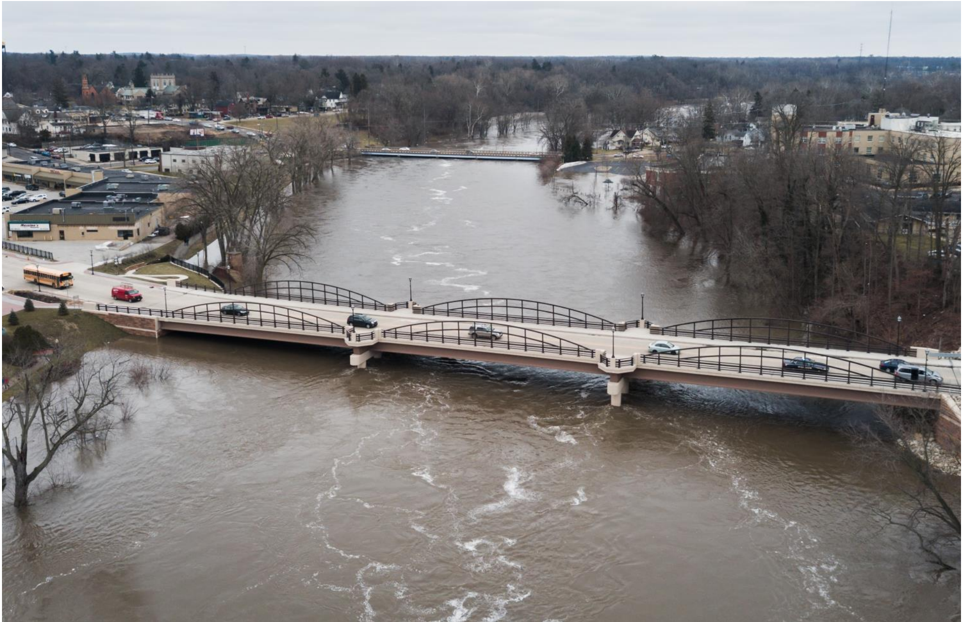
Main Street Bridge (M-139) in Niles during the Flood of February 2018 (Photograph courtesy of Matt Dunlap).
